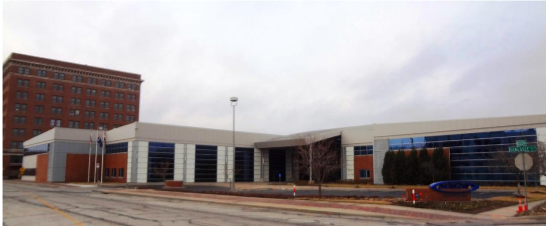
Butler Manufacturing Co. on a 4.5-Acre Brownfield Redevelopment Site, Kansas City, MO
